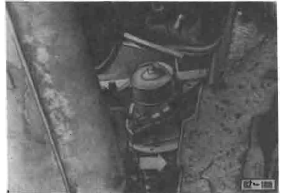
Fig. 16 Air circulation blower, replacing
