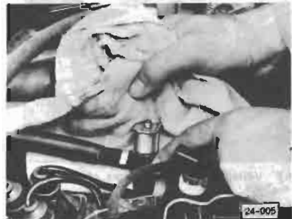
Fig. 3 Cold start valve, checking for leaks
